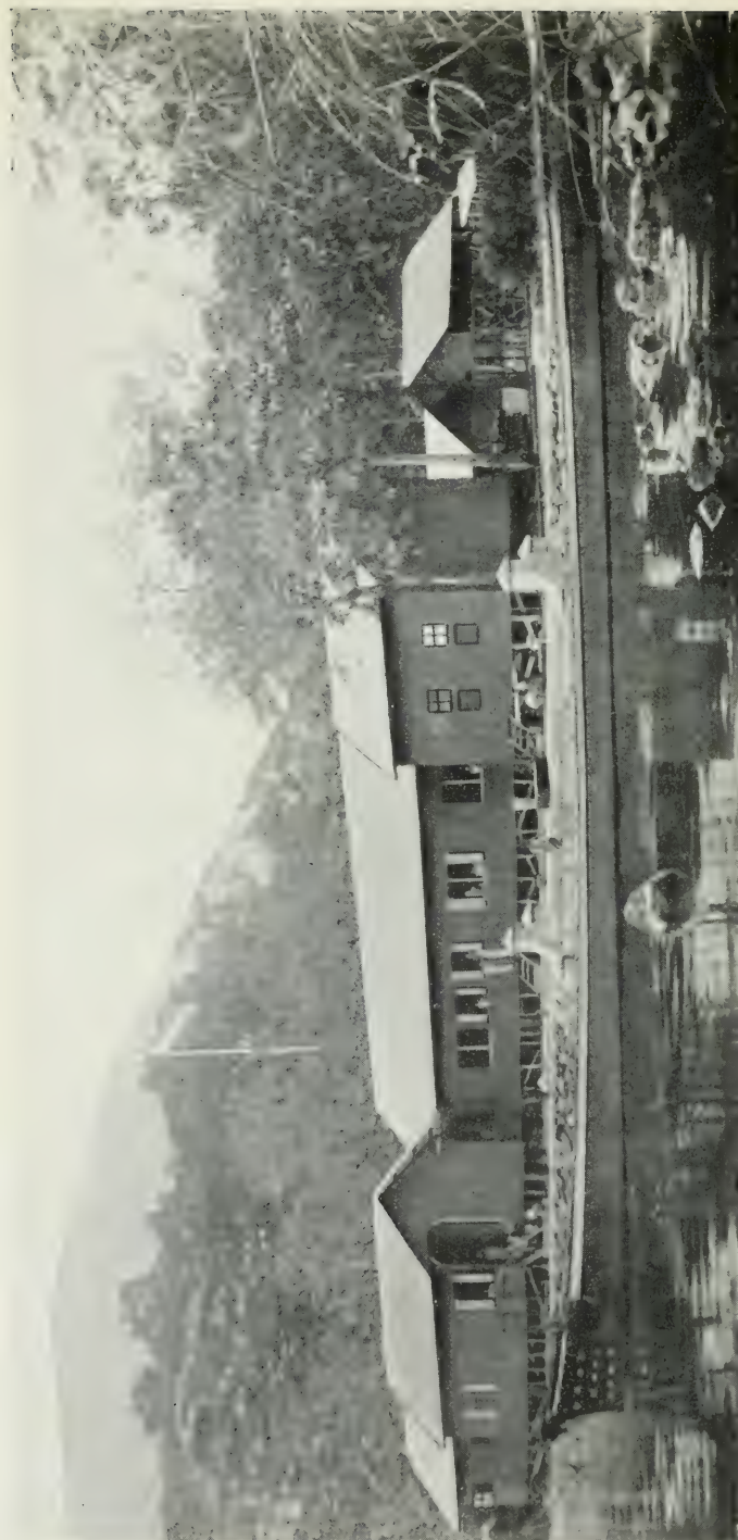
FIG. 113. BUILDING ON PILES: SUMATRA.
